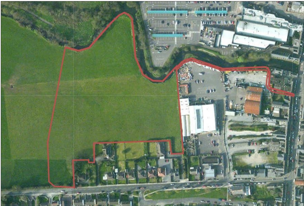
Figure 2: Aerial image depicting the boundaries of the subject application site (red outline)
